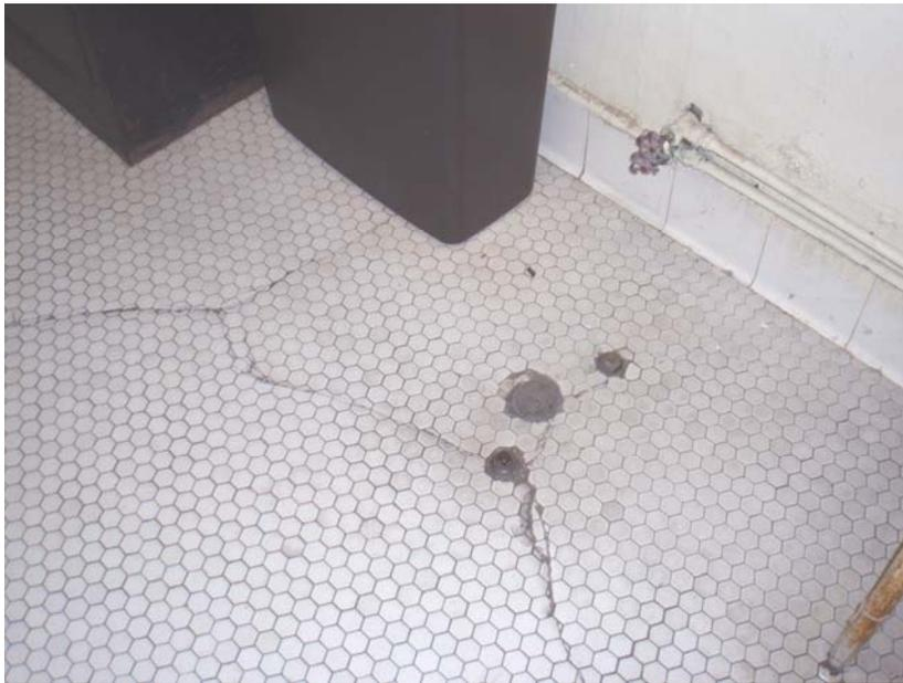
**Photograph No. 3.** Entrance to bathroom at Judith C. White Senior Center showing small pipes protruding from floor, possible tripping hazard
