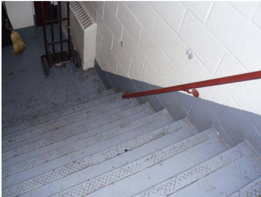
**Photograph No. 2.** Poorly lit exit stairway with broken handrail at the Jackie Robinson Senior Center.
