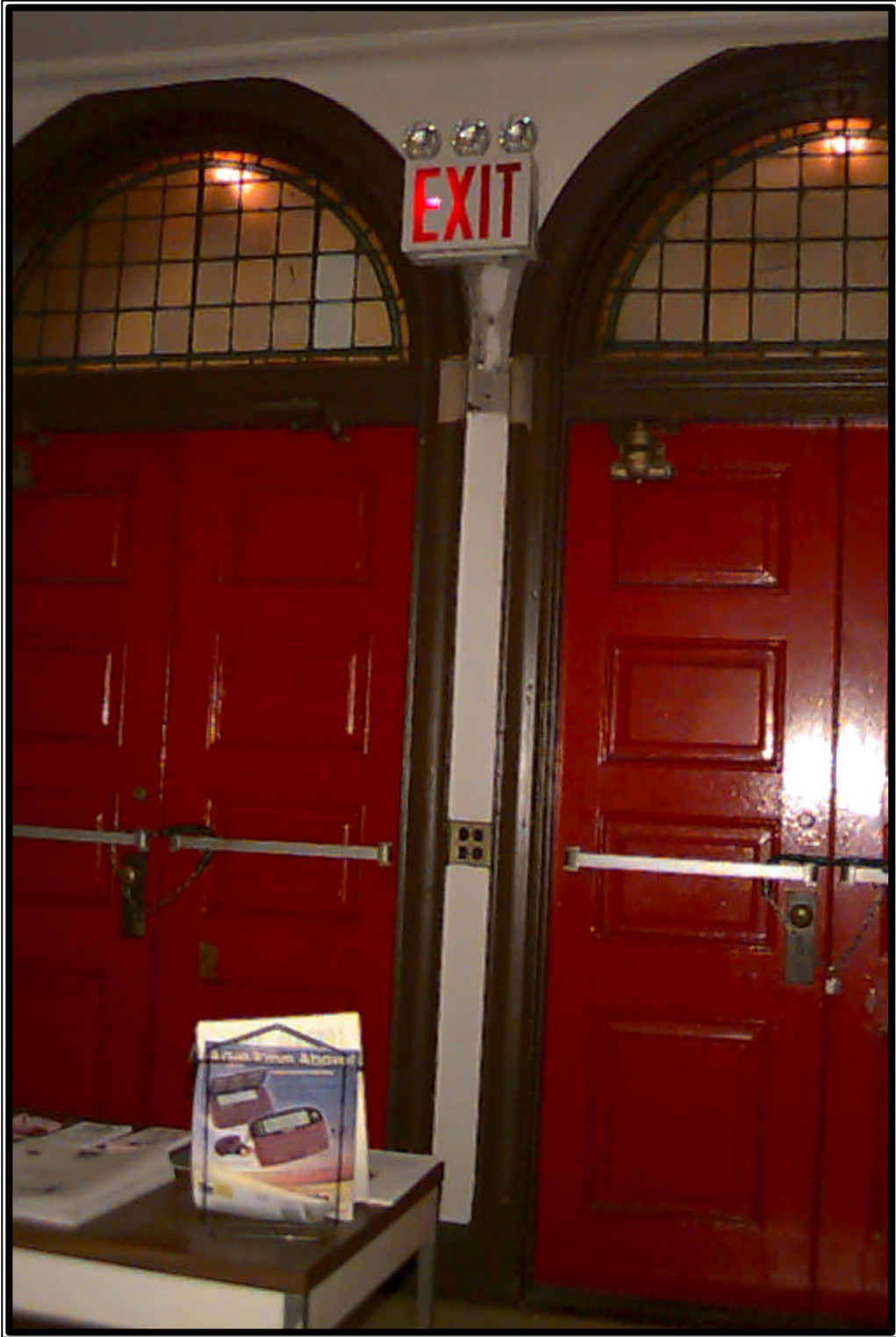
Photograph No. 4, Padlocked exits at Community Lounge Senior Center in Manhattan.
