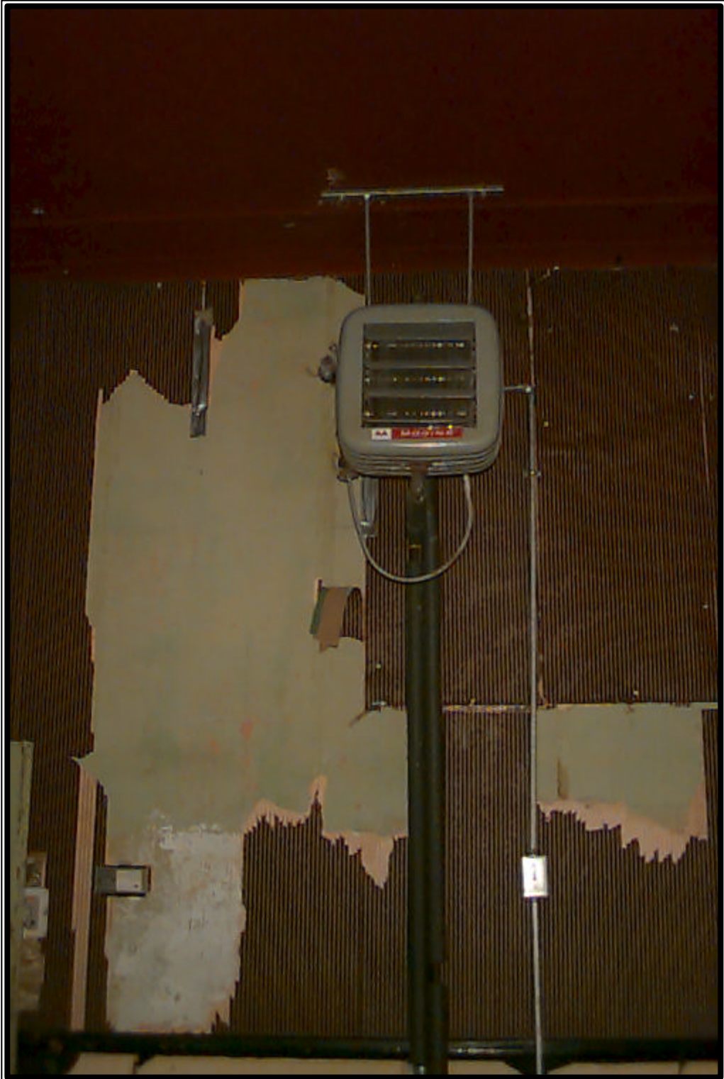
Photograph No. 12 , Damaged wallpaper in a program room at IPR HE Corona Senior Center in Queens.
