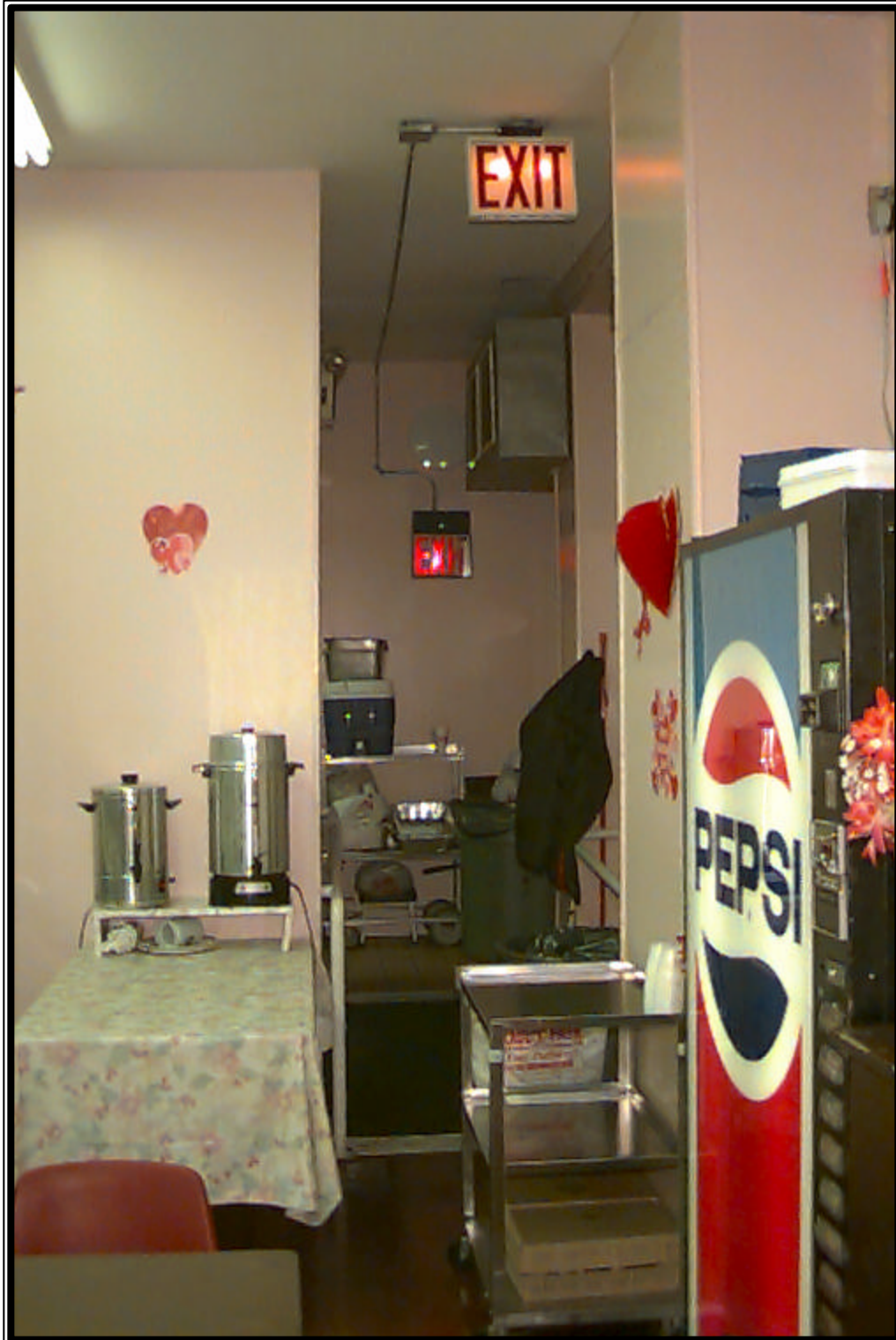
Photograph No. 5 , A partially blocked exitway at Elmcour Senior Center in Queens.
