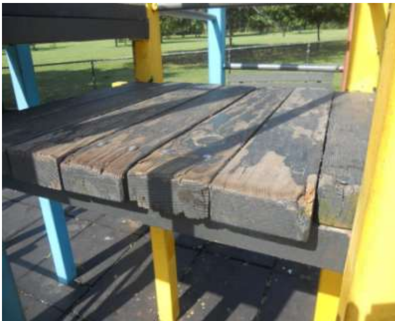
5. Soundview Playground Chipped and peeled paint on play equipment
