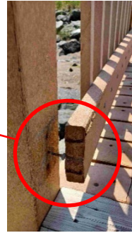
Broken Piece / Disconnected Bottom Rail
