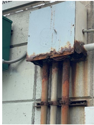
Corroded utility box with exposed electrical wires - open CMR condition flagged by DOT in 2016 (July 2023)
