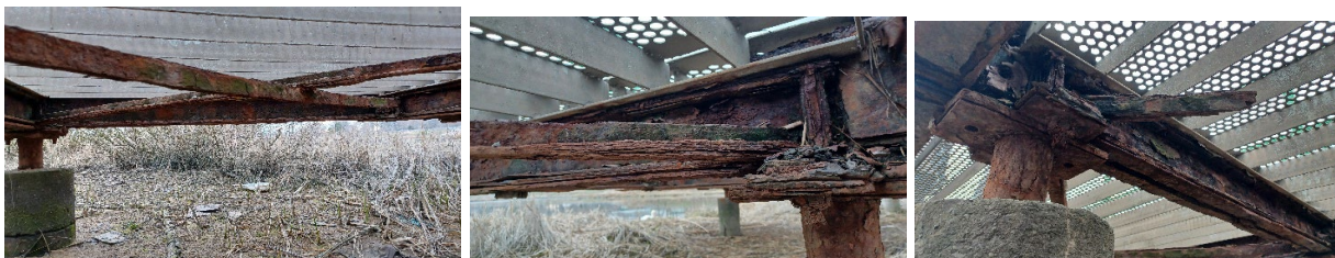
Severe Corrosion in Steel Structure
