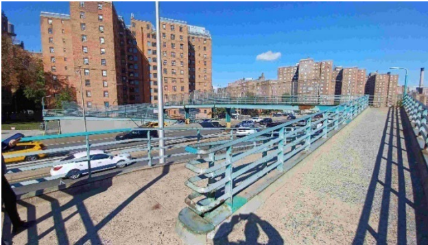
General Bridge View (Looking North)
