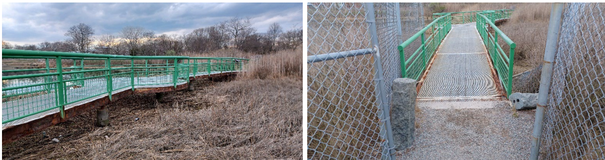
Severe Corrosion in Steel Structure
