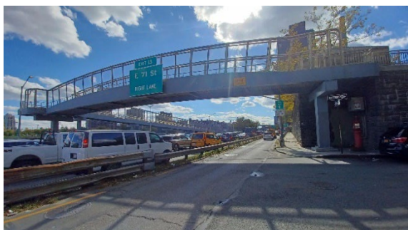
General Bridge View (Looking South)
