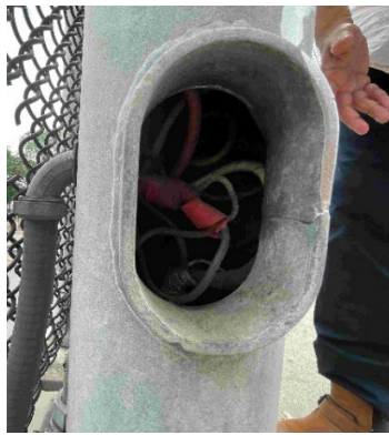
Missing handhole cover with exposed electrical wires – open CMR condition flagged by DOT in 2016 (July 2023)
