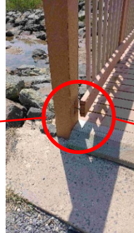
Broken Piece / Disconnected Bottom Rail
