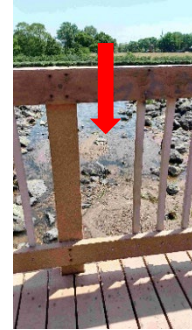
Missing Spindle
