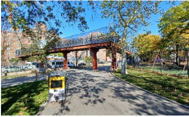
View of bridge looking north
