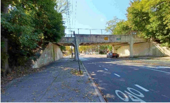
General Bridge View (Looking West)
