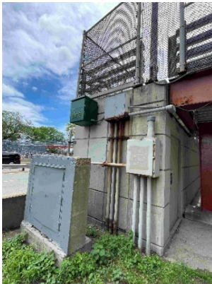
Corroded utility box with exposed electrical wires - open CMR condition flagged by DOT in 2016 (July 2023)
