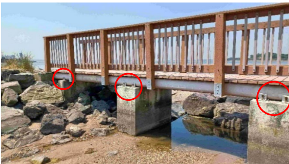
Horizontal Bolt Heads Intact (Entire Park Side Except Far Right – Not in Photo)
