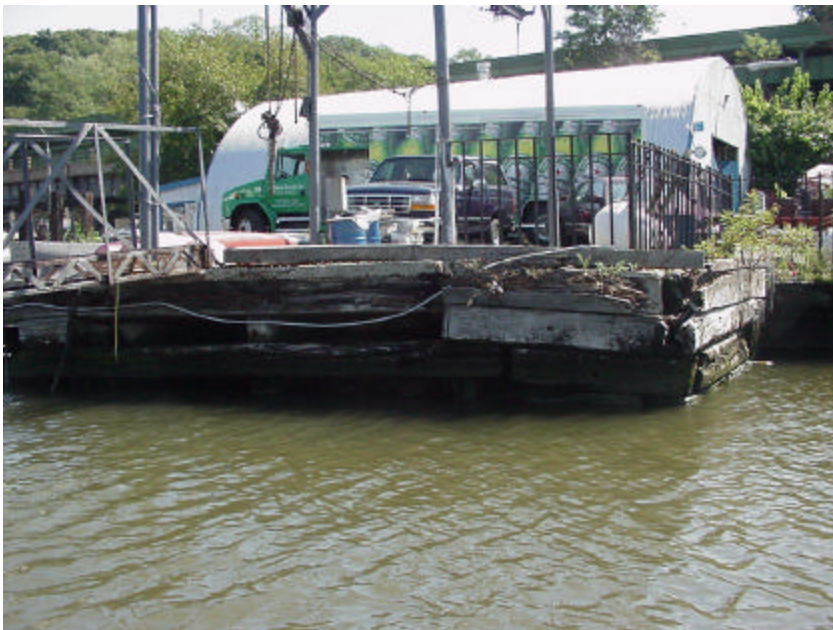
This photograph and the next one shows that the bulkhead is settling. This stationary pier provides access to the floating dock.
