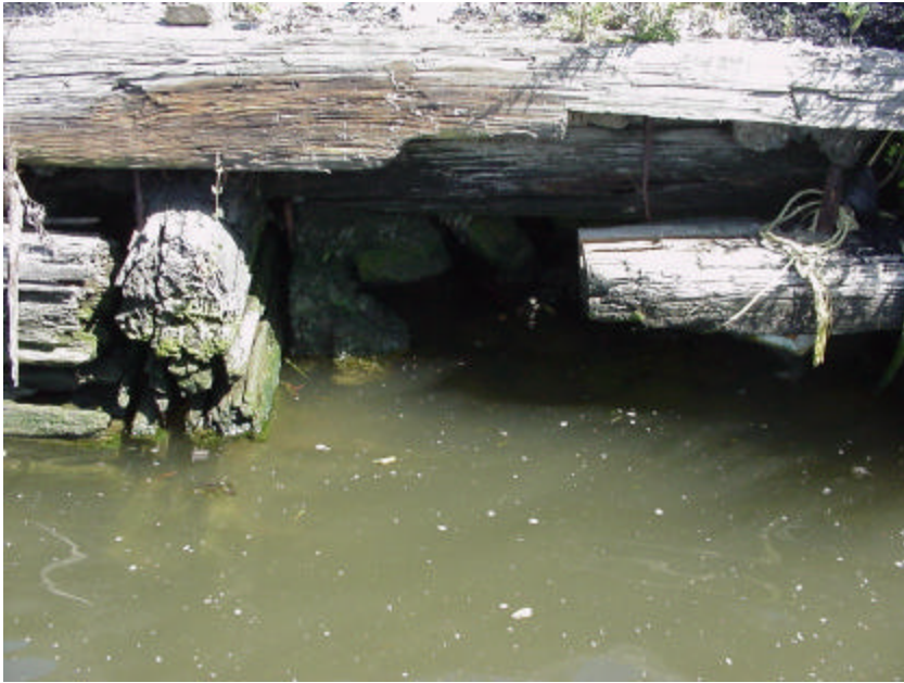
The rotting bulkhead beneath the stationary pier.
