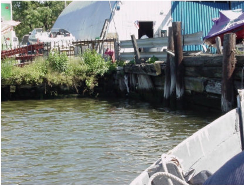
Another view of the bulkhead showing deteriorated beams and underlay.
