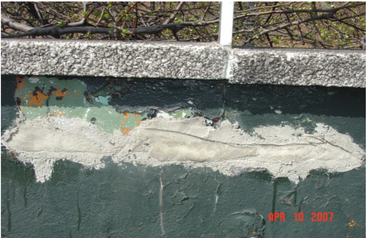
Lasker Rink – Picture # 2: Damaged Parapet Wall
