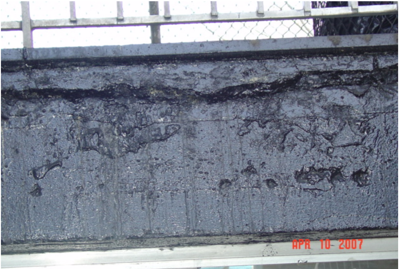
Lasker Rink – Picture # 5: Chipping/Separation of the Concrete Surface on the Upper Deck
