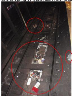
Similarly, we observed a vacuum train in operation on one track at the 14th Street/8th Ave station on the A train line and found that most of the trash also remained on the track bed after the operation of the vacuum train. (See Appendix II, page 3 for pictures of debris found before and after this station was cleaned by the vacuum train.)
