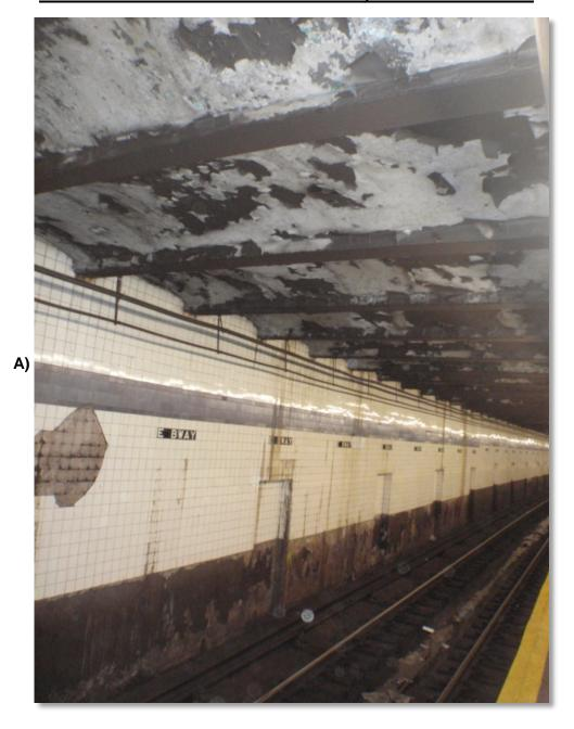
A) Excessive peeling paint on ceiling over track. (Photo taken on 3/14/14)
