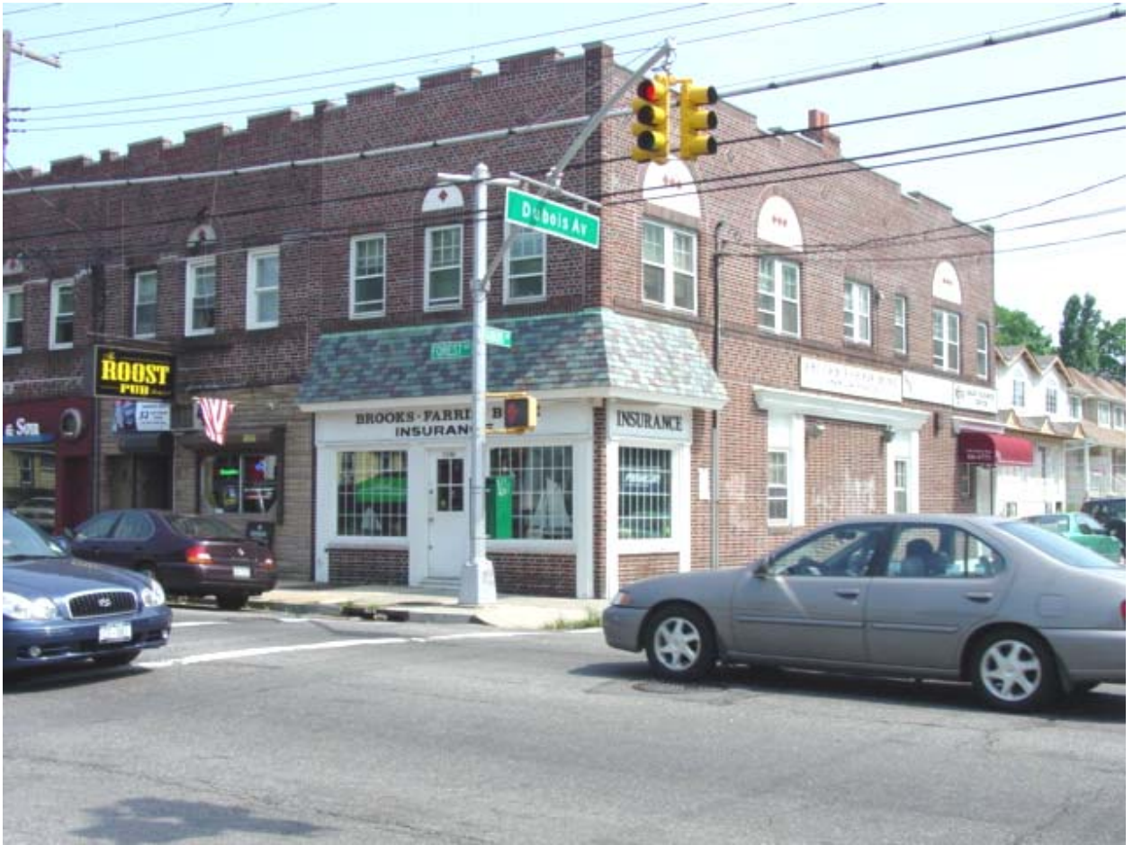
1146 Forest Avenue: Finance records inaccurately listed this property as a “Primarily One-Family with One Store or Office” (Tax Class 1, Building Code S1).
