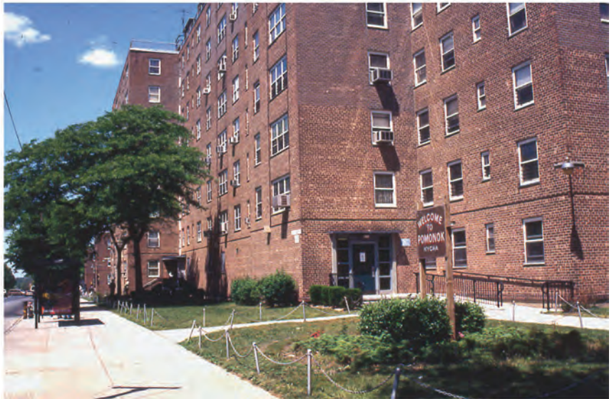
Pomonok Houses, Queens
