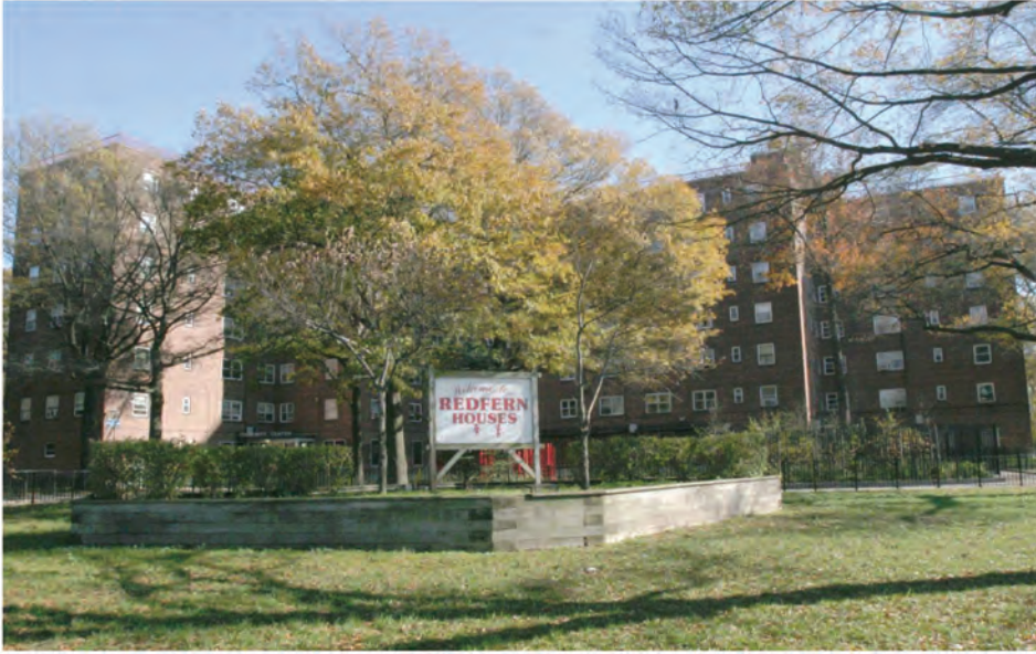
Redfern Houses, Queens
