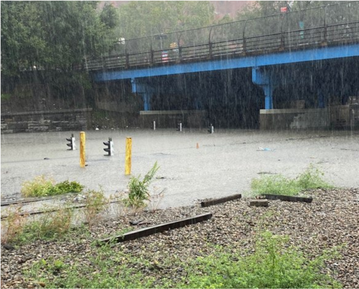
Figure 5: Flooded Mott Haven Yard, Metro-North Railroad 32
