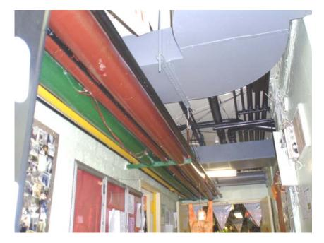
**Photograph No. 9.** Overhead pipes covered in red and green plastic; and exposed vents and wires at the Boulevard Senior Center.
