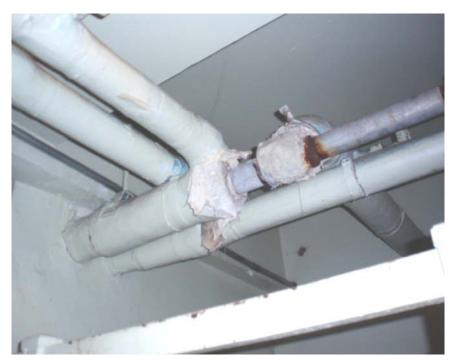
**Photograph No. 6.** Possible asbestos pipe insulation that appears to be damaged and friable at Kennedy/Central Harlem Senior Center.
