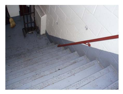
**Photograph No. 2.** Poorly lit exit stairway with broken handrail at the Jackie Robinson Senior Center.
