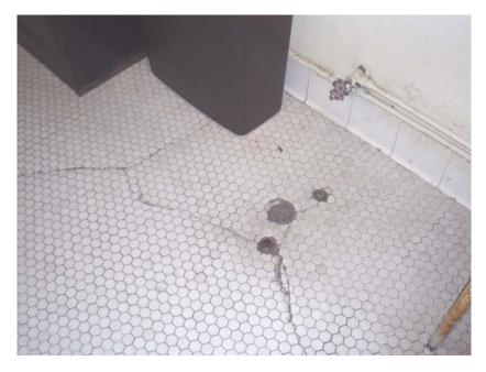
**Photograph No. 3.** Entrance to bathroom at Judith C. White Senior Center showing small pipes protruding from floor, possible tripping hazard
