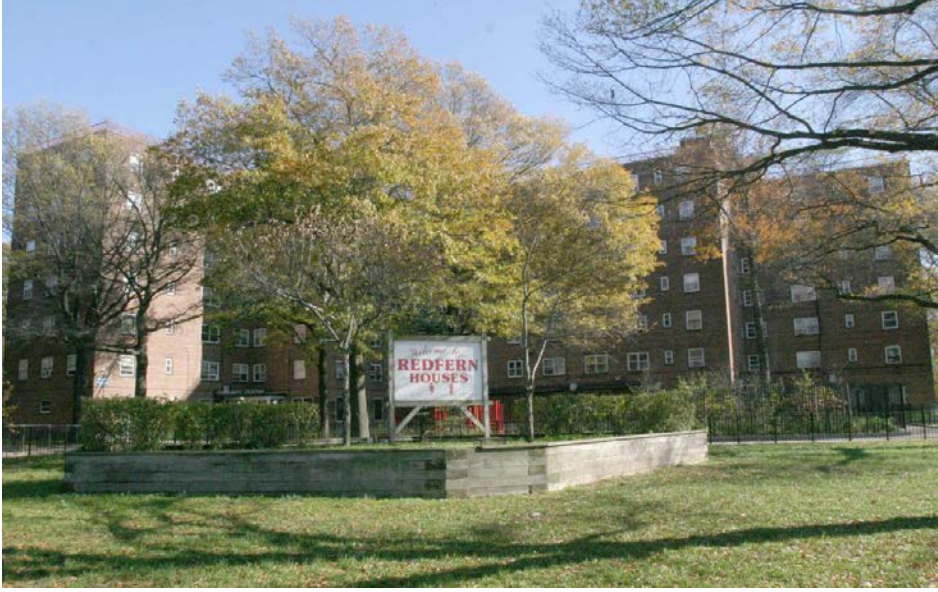
Redfern Houses, Queens
