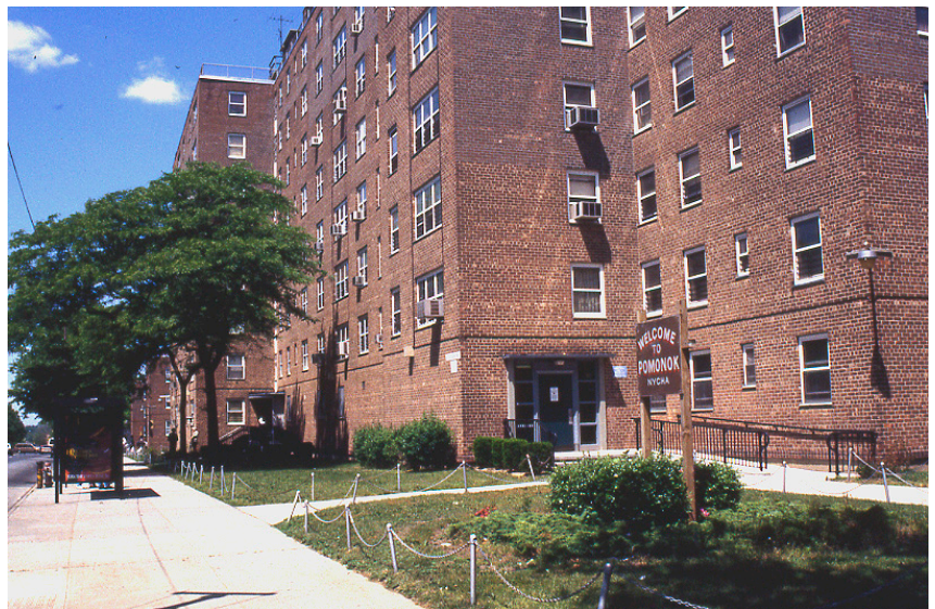
Pomonok Houses, Queens
