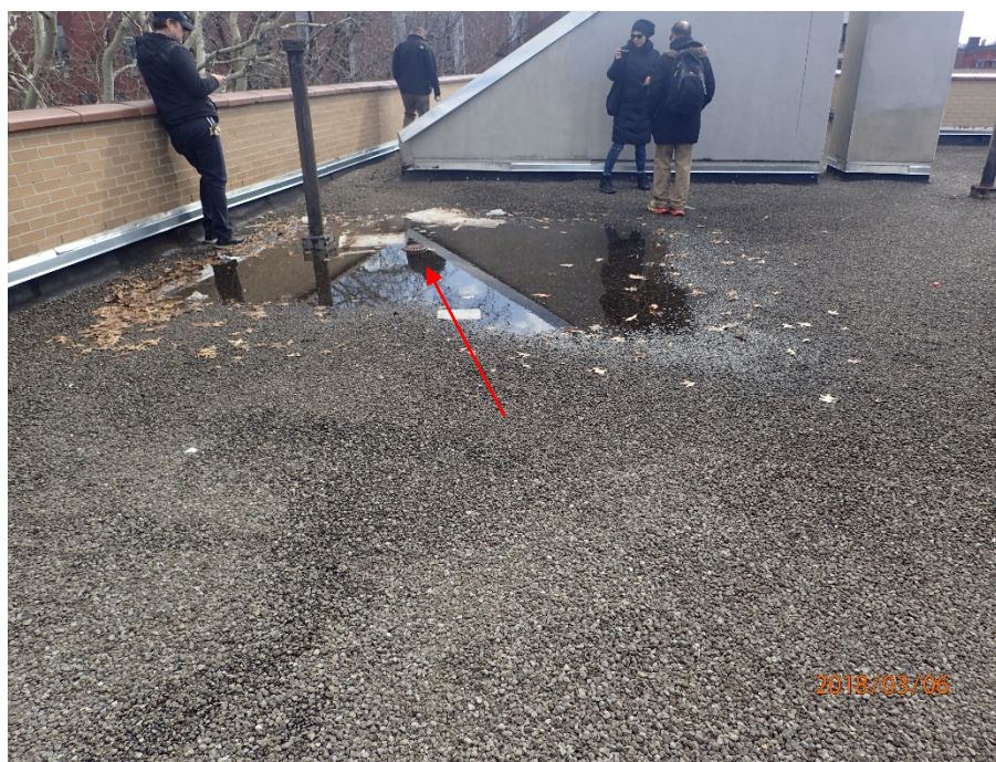
Williamsburg (Bldg. #13); 171 Scholes St, Brooklyn Clogged Drain and Debris
