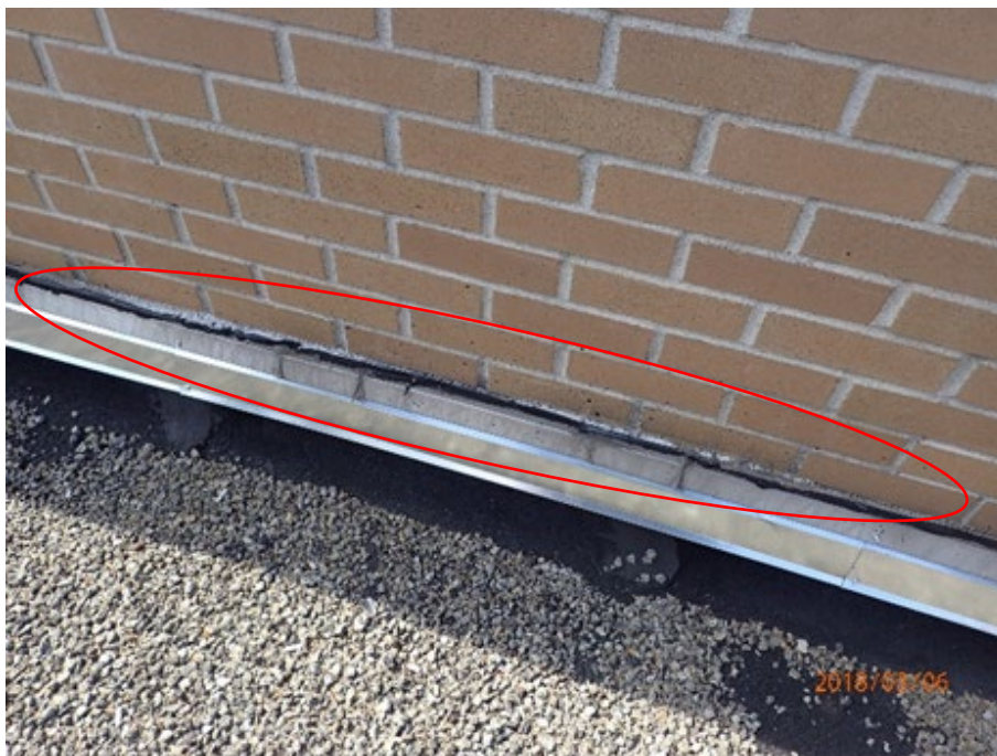
Williamsburg (Bldg. #13); 171 Scholes St, Brooklyn Clogged Drain and Debris
